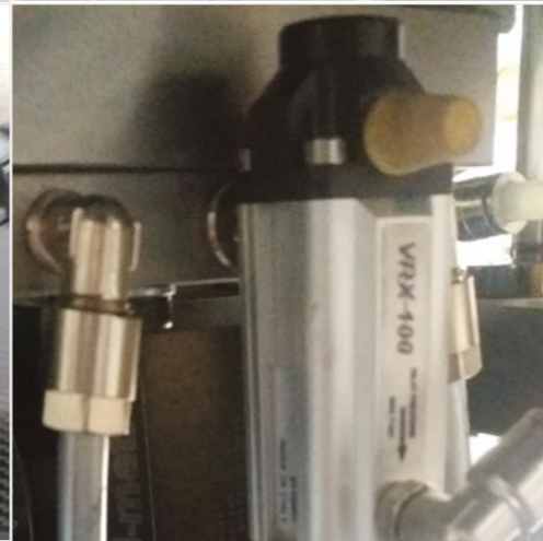
Cooling of control cabinets
