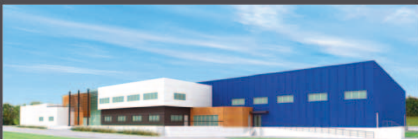
New offices with High Quality Environmental standards
